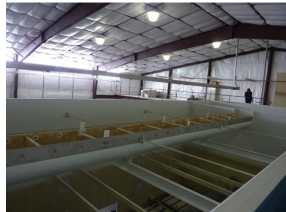
Figure 2.3-3. Photograph of the Existing Water Treatment Plant
