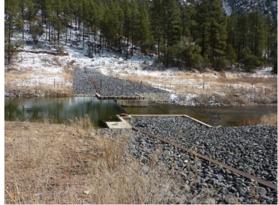
Figure 2.3-2. Photograph of the Existing Diversion Dam
